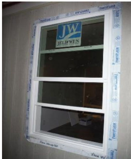
Figure 8 Flashing at sides and top of window
