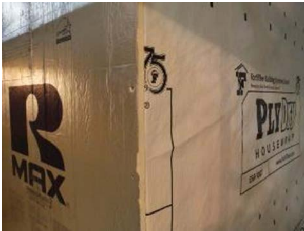
Figure 6. Foam sheathing over house wrap
