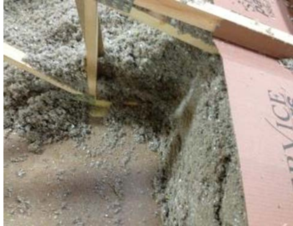
Figure 10. Insulation fills eave area without voids
