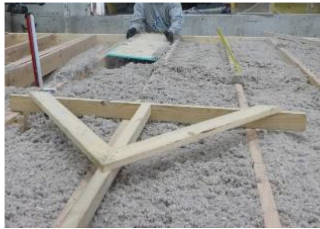
Figure 5. Insulation “presettled” and raked flat
