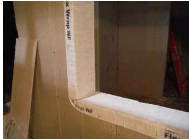
Figure 7. Flashing on sill and sides of openings
