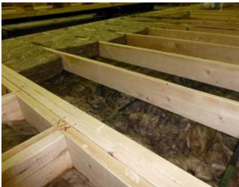
Figure 2. Insulation in progress, shows blankets below floor framing
