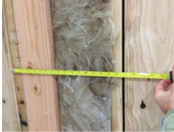
Figure 12. Lay-flat studs for mounting DHP compressor
