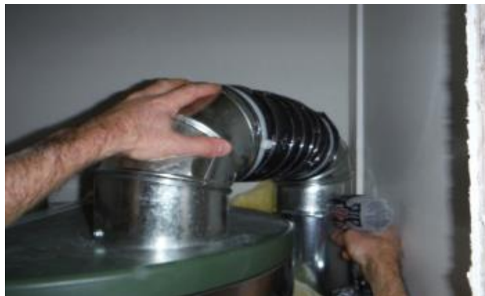
Figure 16. HPWH intake duct connection
