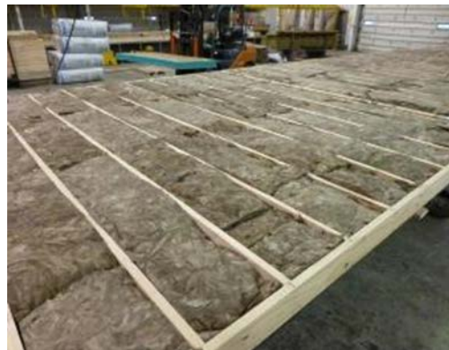
Figure 3. Fully insulated floor
