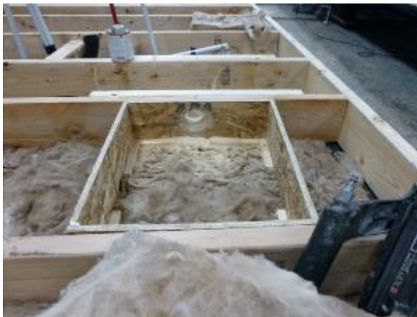
Figure 4. Blanket below framing, boxed-in utilities
