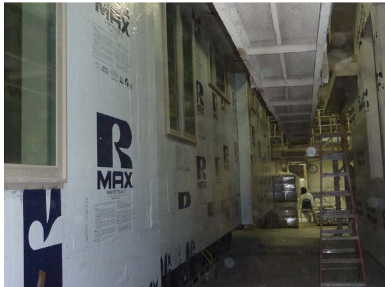
Photo 1. Rigid foam sheathing on walls
