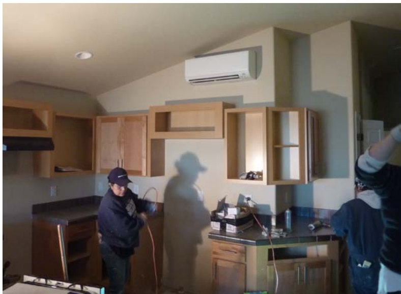
Photo 3. DHP indoor head installed in plant
