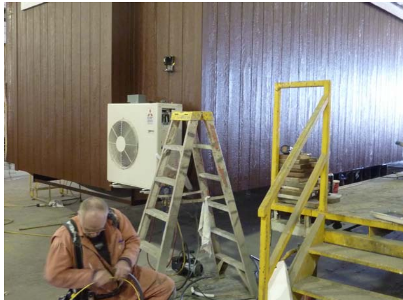
Photo 2. DHP compressor being installed in the plant
