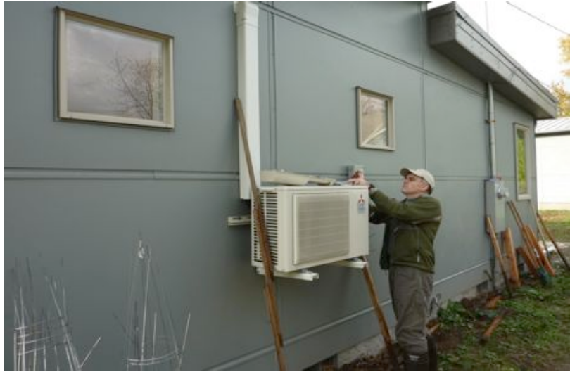
Figure 6. Installing sensors on the Portland site DHP
