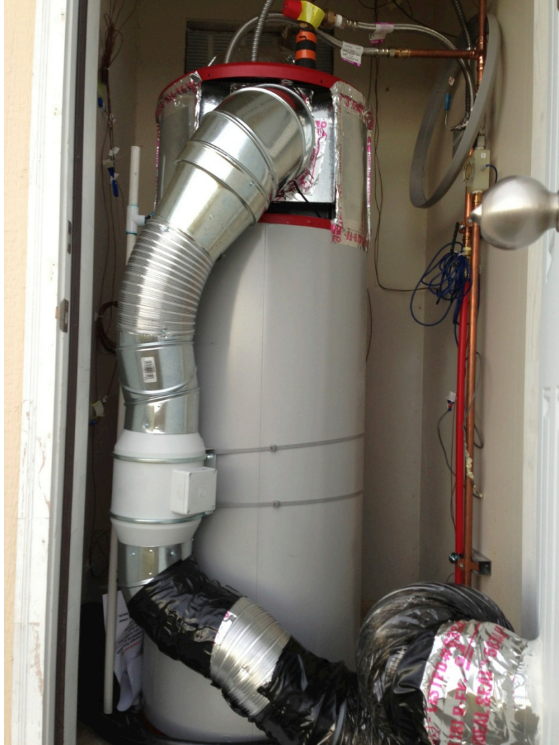
Figure 16. HPWH modifications to allow fully ducted operation
