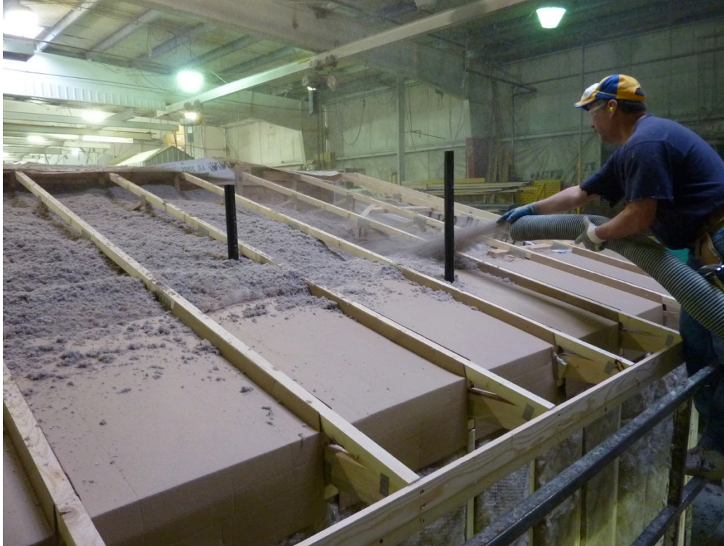
Figure 9. Transition to blown-in insulation for deeper attic cavity area
