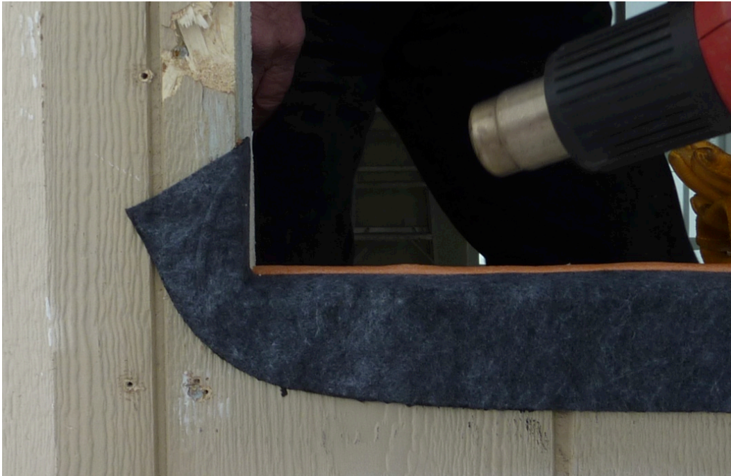
Figure 5. Flexible flashing window sill pan
