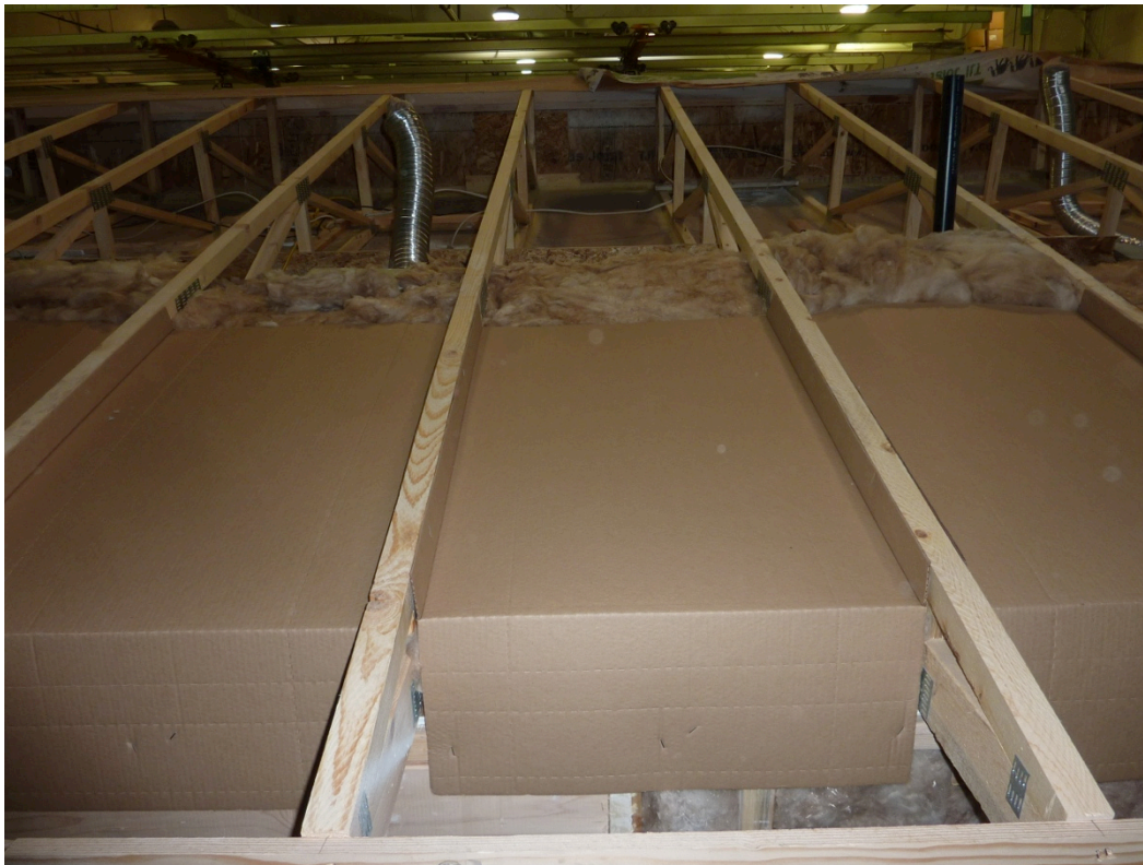
Figure 8. Compressed R-38 batts with baffles at eaves
