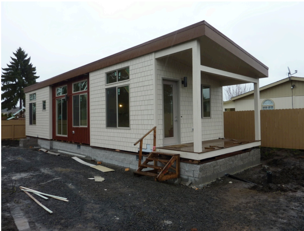
Figure 4. Exterior foam-sheathed home after transport
