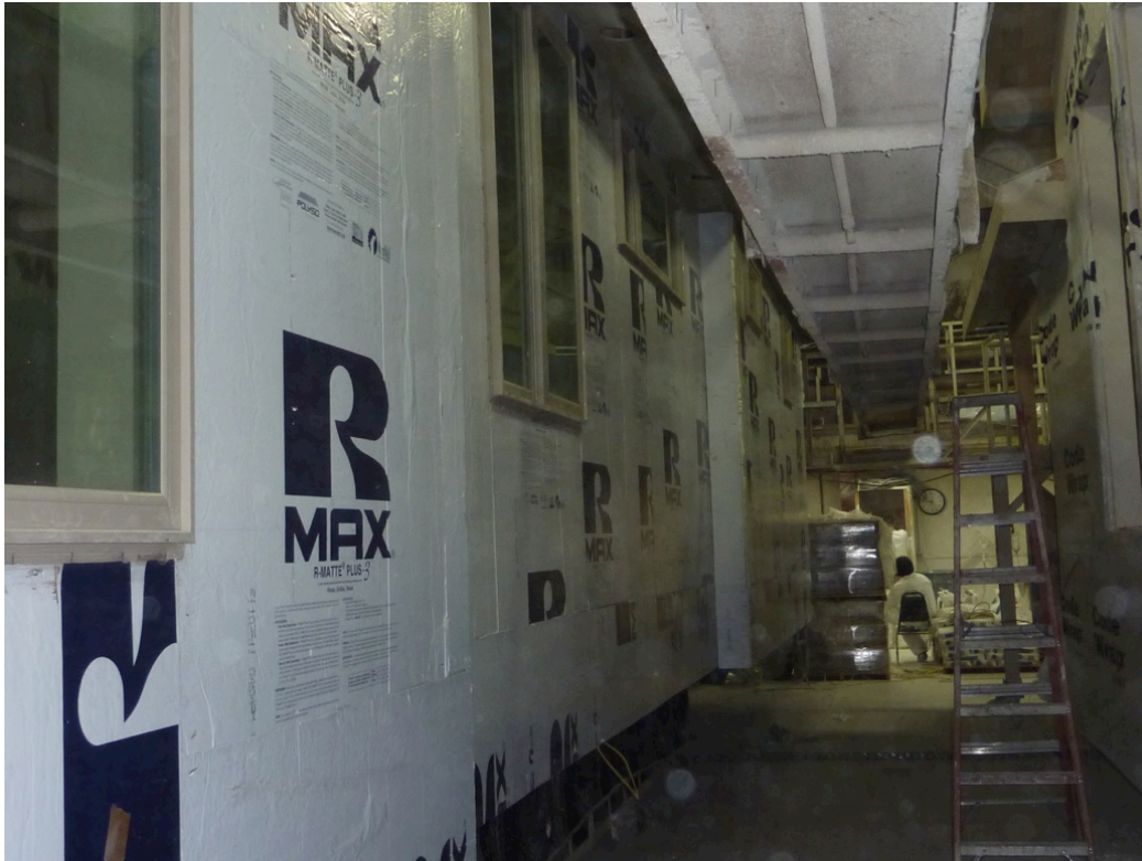
Figure 3. Exterior foam installed
