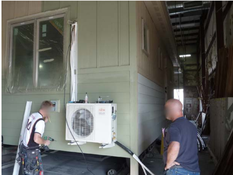
Figure 13. DHP compressor on end wall with indoor head on other side of wall—“up and in” installation
