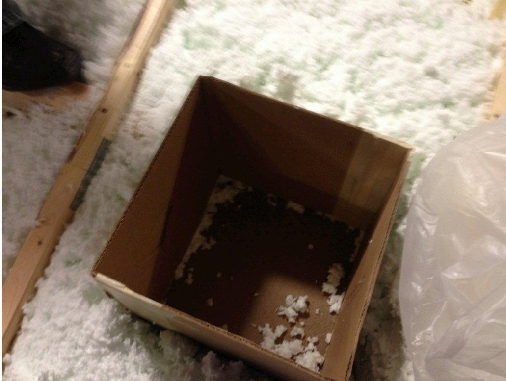
Figure 11. Core sampling of dense-packed insulation
